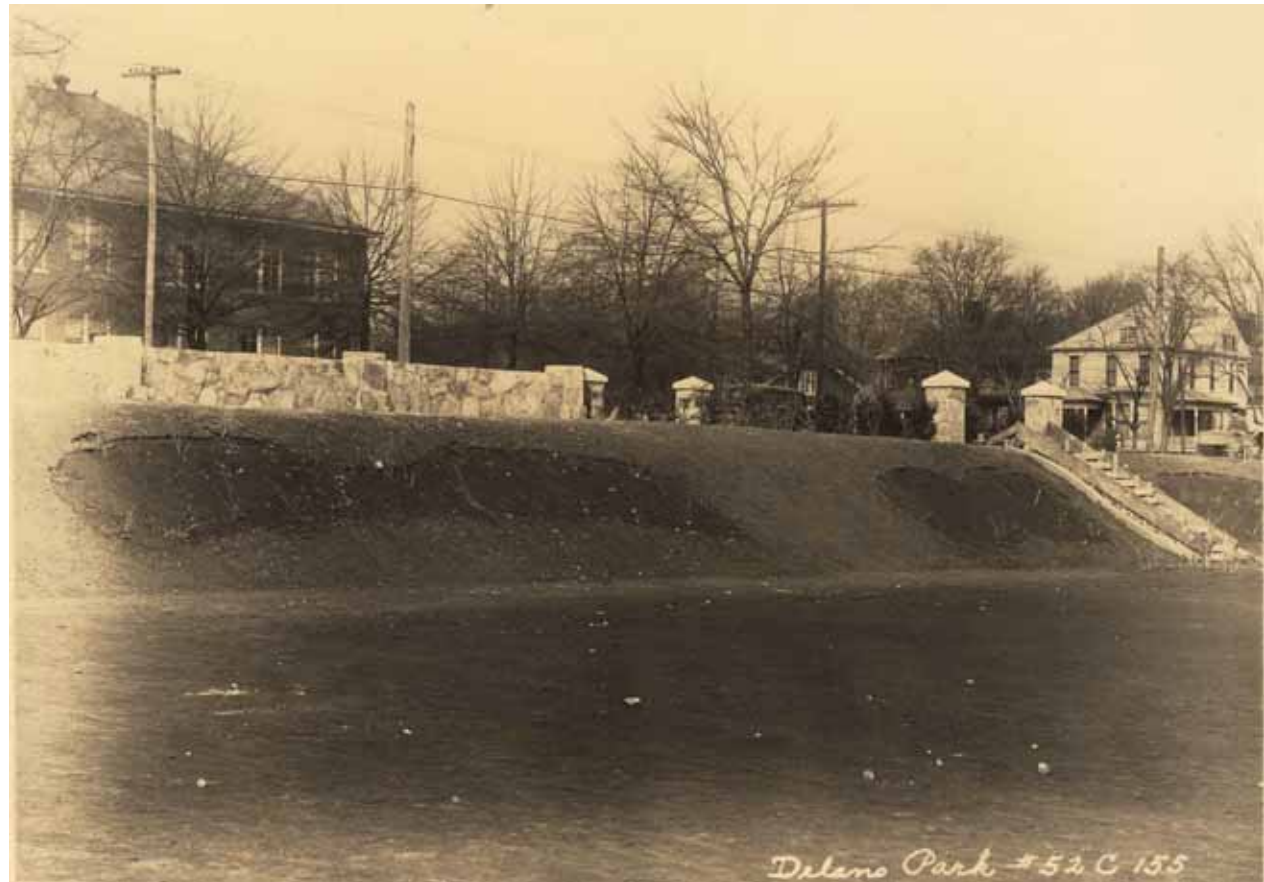
4 th Avenue Stars, Plantings and Sports Field (Armory Site)
